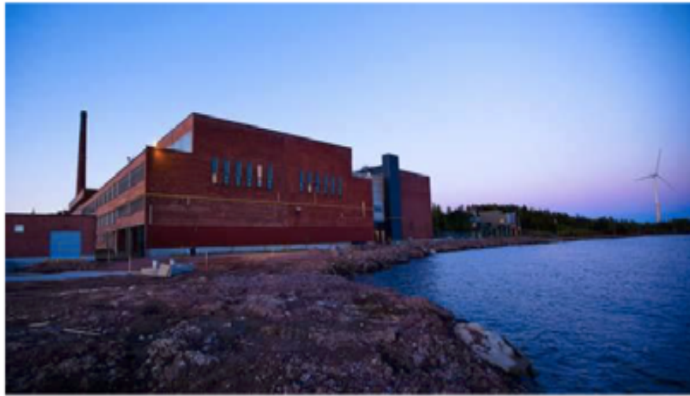
A Google data center in Hamina, Finland, is housed in a former paper mill.
